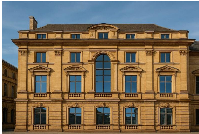
An Example of Window Film for Heritage Buildings.
